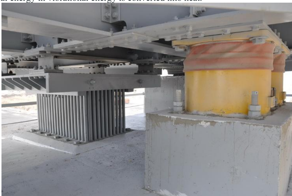
Figure 2. Seismic protection devices made of shock absorbers.
