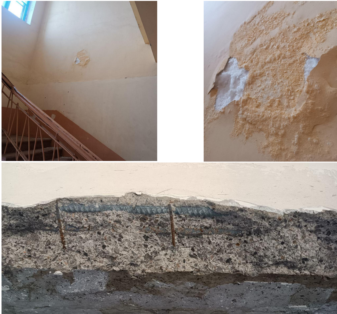
Figure 3. Influence of the aggressive environment on the structures of multi-story residential buildings.
