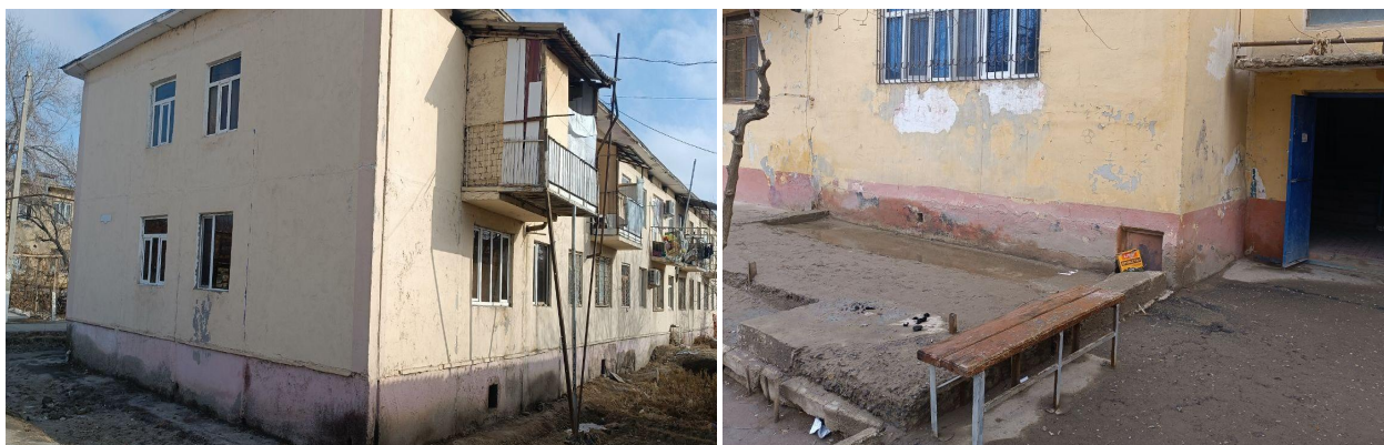
Figure 2. Soaking of the foundation of an apartment building after rainfall.
