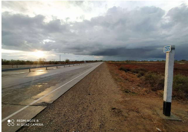
Fig. 1. Section of the A-380 Highway crossing the desert territory of the Republic of Karakalpakstan.
